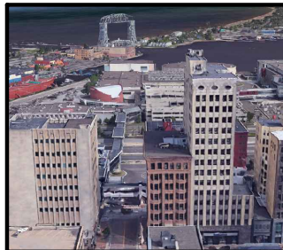
Lonsdale Building Location
