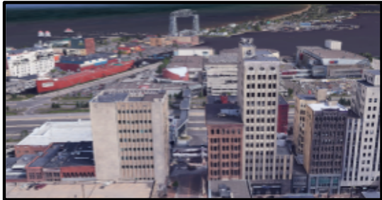
Lonsdale Building Location
