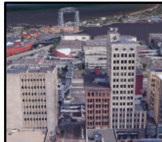
Lonsdale Building Location
